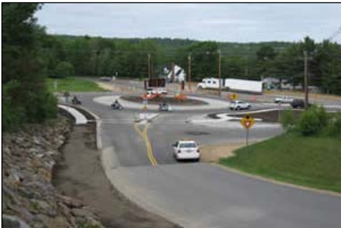
US 3/Parade Road Roundabout Construction (NHDOT)
